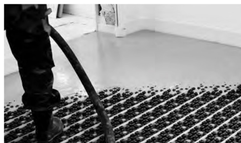
Flooding the underfloor heating system self-leveling mass.
