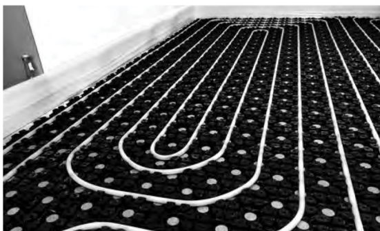
Underfloor heating installation with usage of LOWTOP castellated mat.
